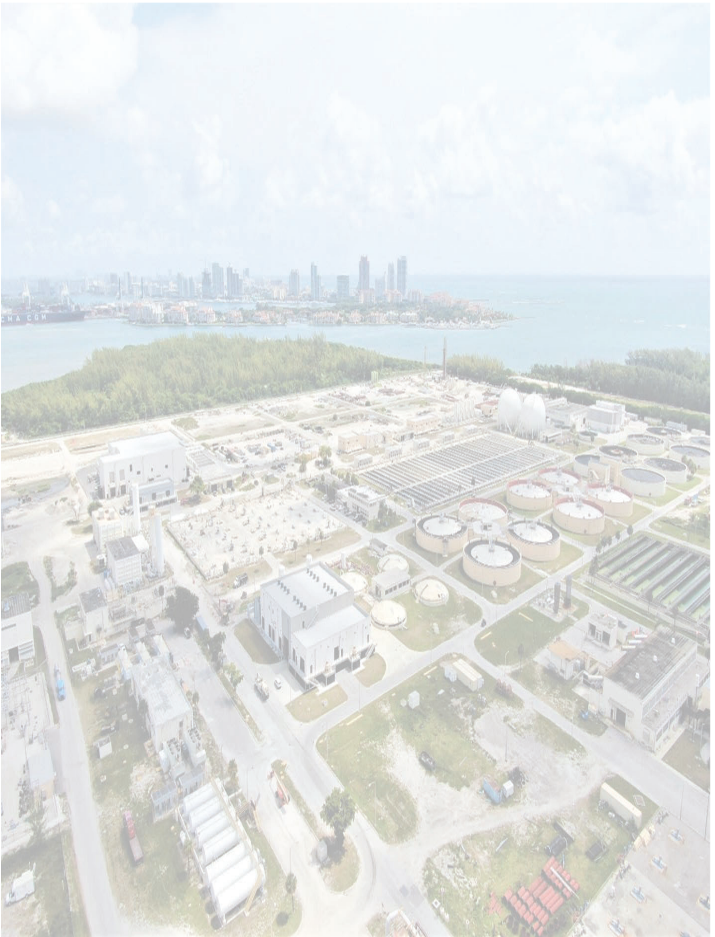
The cover's design is an aerial view of the Central District Wastewater Treatment Plant.
