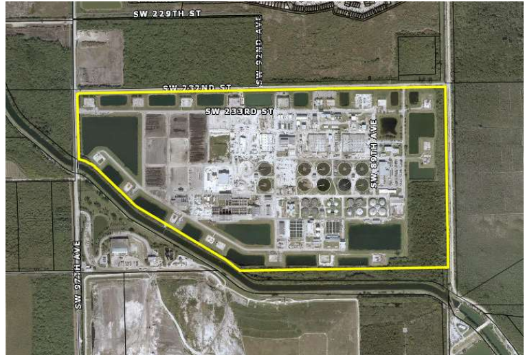
South District WWTP (Courtesy MDPA)
